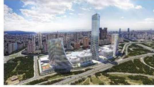
Metropol İstanbul - 1,719 flats/pisos
